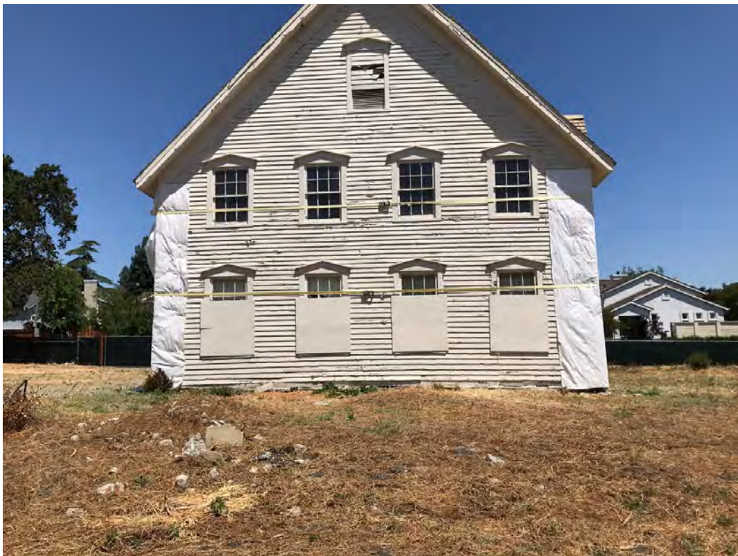
Photo 16 – View of house, looking north from south fence
