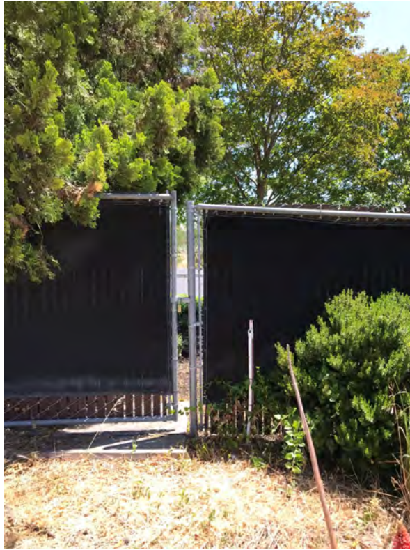
Photo 19 – Stubbed PVC pipe, near east gate
