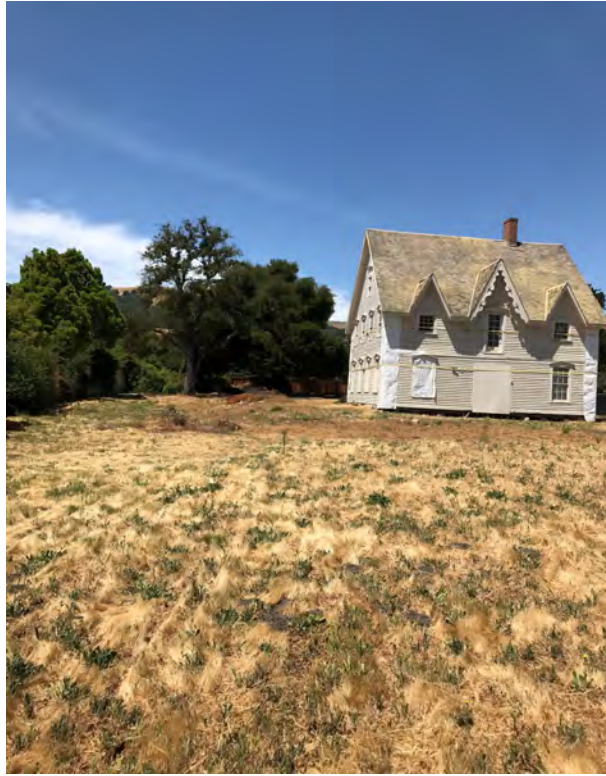
Photo 17 – View of house, looking west from east fence
