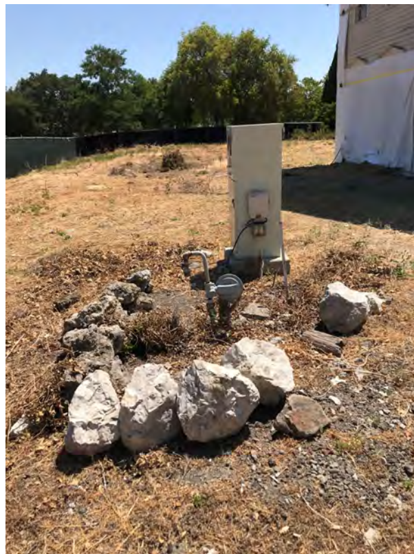
Photo 12 – Center of site, looking east, utility connections
